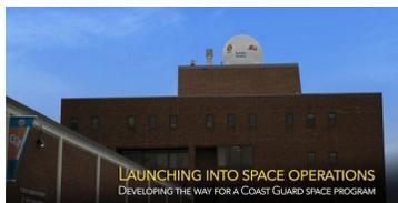
The satellite communications ground station sits on the roof of Smith Hall at the U.S. Coast Guard Academy in New London, Conn. The main feature inside the radome is a 3-meter dish antenna and communications components. It is helping to launch the Coast Guard into **an era of space operations**.
