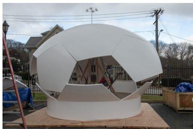
includes sites in Dayton, Ohio; Monterey, California; and Logan, Utah, for frequent contact opportunities with two Polar Scout CubeSats, named Kodiak and Yukon in Low Earth Polar Orbit. The most visible element is the 18-foot diameter fiberglass radome on the roof of Smith Hall. It houses a 3-meter dish antenna controllable in azimuth and elevation so it can automatically point towards the satellite during a pass. The radome also houses the
