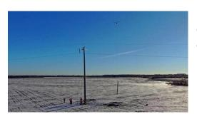
FulcrumAir is pleased to announce that it is now offering slinging operations to assist in powerline construction and maintenance, utilizing its E7500 heavy lifting UAS. Work was recently done with K-Line Line Maintenance and Construction on a 138KV line being reconstructed for one of the leading power providers in Canada.
