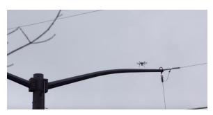
Already accustomed to using <u>drones to inspect</u> its enormous 1,400 circuit miles of transmission infrastructure, the <u>New York Power</u>
