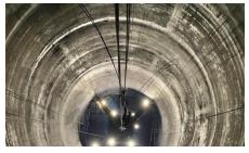
Inspection experts from PIT were recently asked to conduct an internal inspection of a coke drum at an oil refinery in Texas, US, without using scaffolding. Scaffolding is expensive and time-consuming to put up and take down. Inspectors from PIT proposed using a a combination of drone technology and manned rope access within the coke
