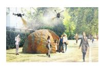
A French architect has showcased an experimental project in which drones spray layers of a mud mixture onto prefabricated frames, rapidly resulting in habitable structures suitable for emergency housing.
