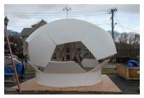
includes sites in Dayton, Ohio; Monterey, California; and Logan, Utah, for frequent contact opportunities with two Polar Scout CubeSats, named Kodiak and Yukon in Low Earth Polar Orbit. The most visible element is the 18-foot diameter fiberglass radome on the roof of Smith Hall. It houses a 3-meter dish antenna controllable in azimuth and elevation so it can
